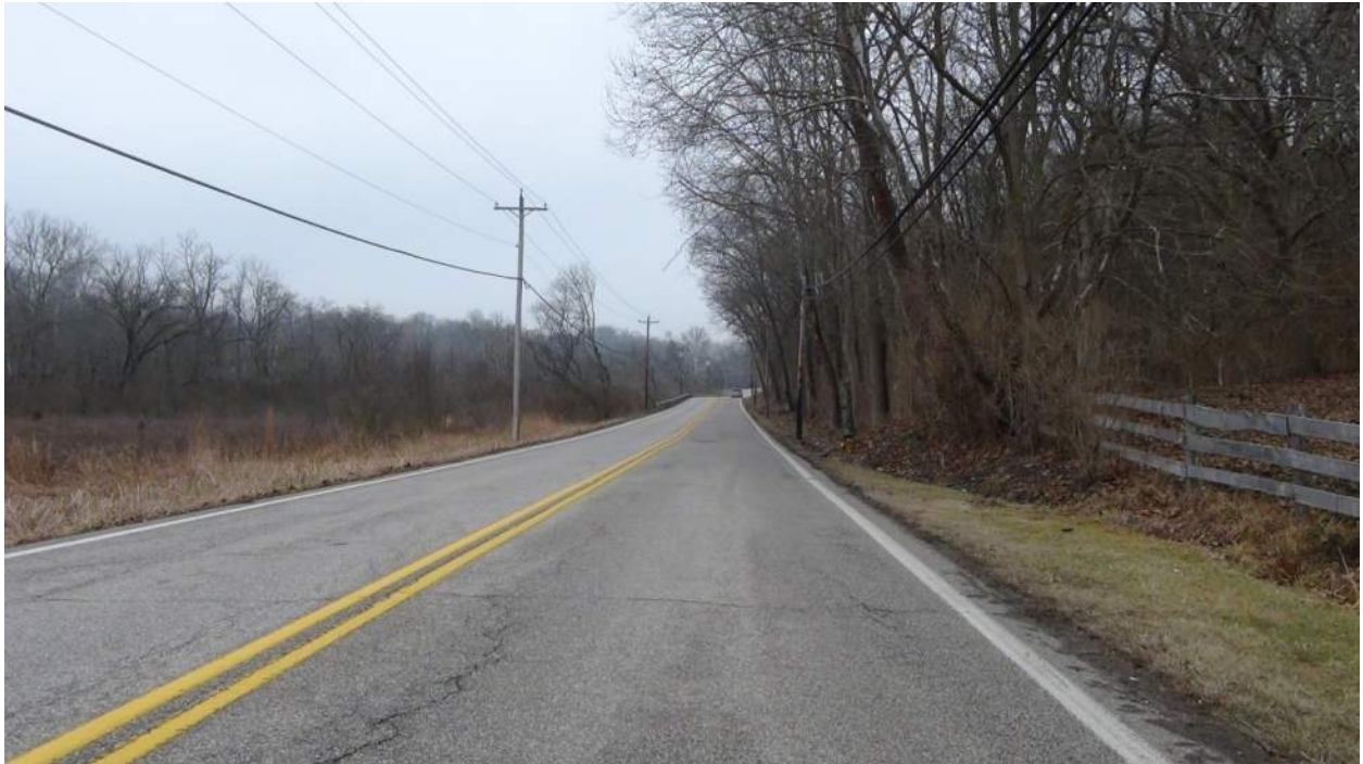
Vehicle making a left turn into driveway continuously seeing a vehicle approaching from the opposite direction (SIGHT DISTANCE – 920 FT)
