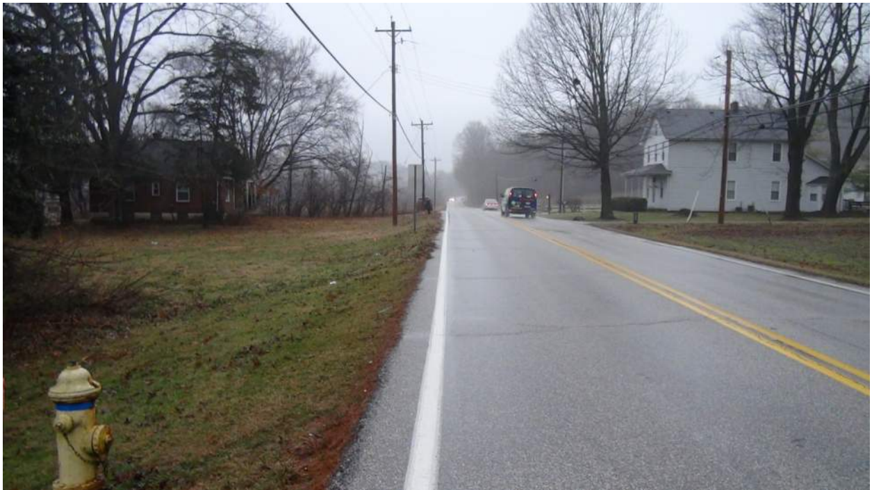
Vehicle making a left turn into driveway continuously seeing a vehicle approaching from the opposite direction (SIGHT DISTANCE - >1000 FT)
